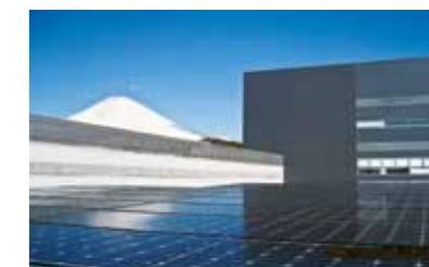
Solar Power Generation Equipment
